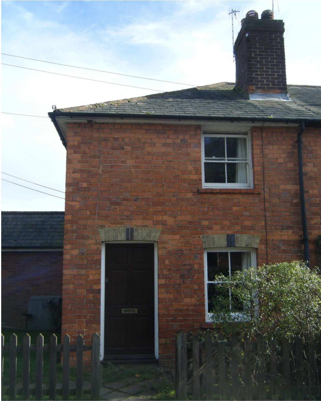
20. Unassuming 19 th C. cottage in Long Barn Road
